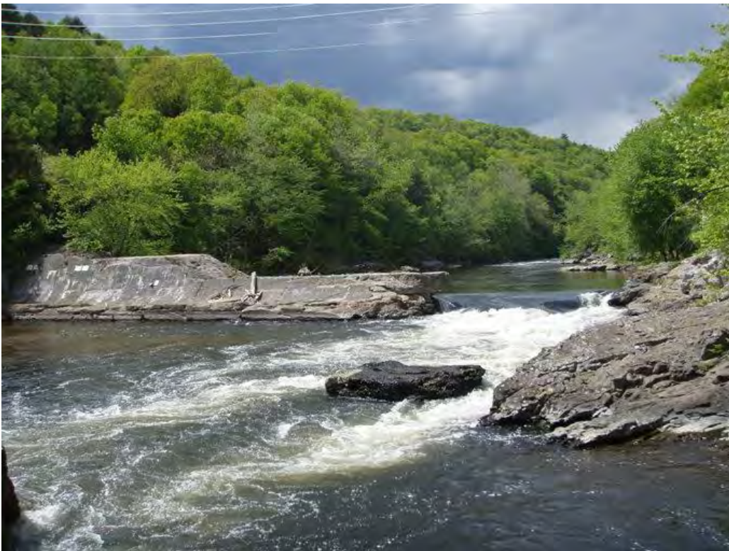
Spoonville Dam on the Farmington River (CT) prior to removal.
