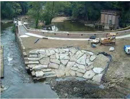
The Kent Dam Restoration, with Bypass under Construction (from ODNR)
