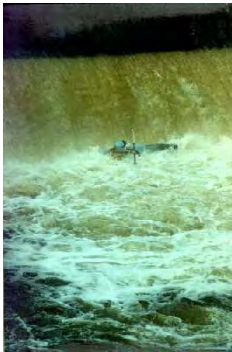
Soon, this hydraulic will be gone.
